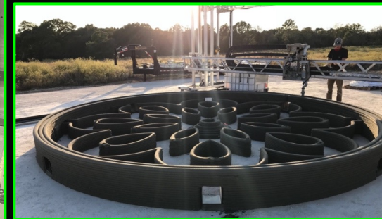
Terrestrial printing of cementitious material
