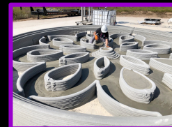
3D Printing w/ Lunar Concrete
